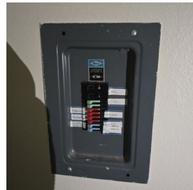
Cordillera Apartments, Chico – Electric Panels slated for replacement
