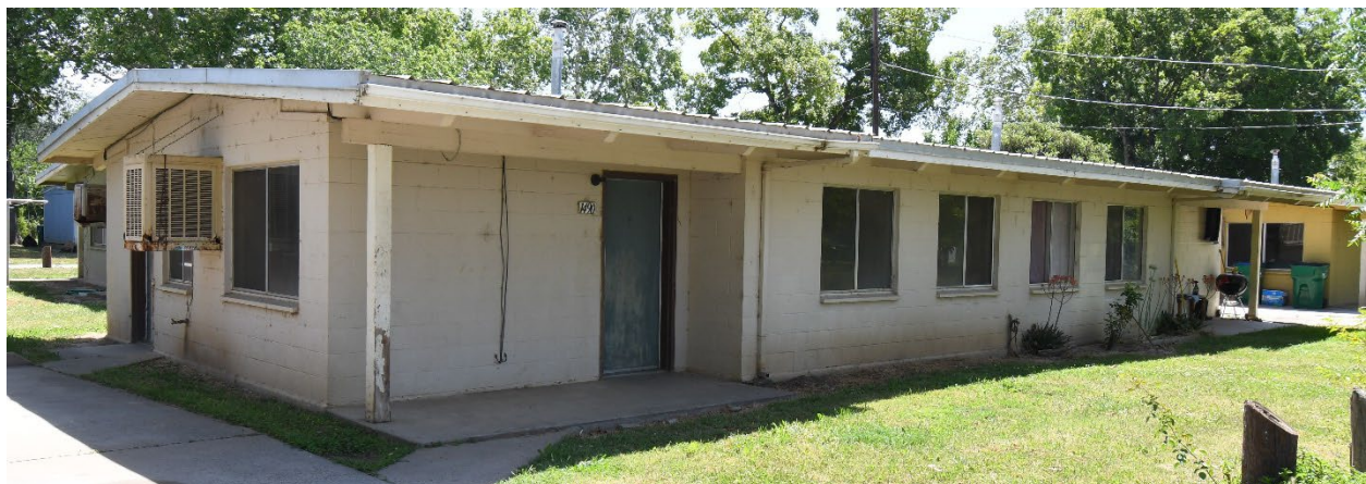
Unrenovated 1980's era Concrete-block Unit
