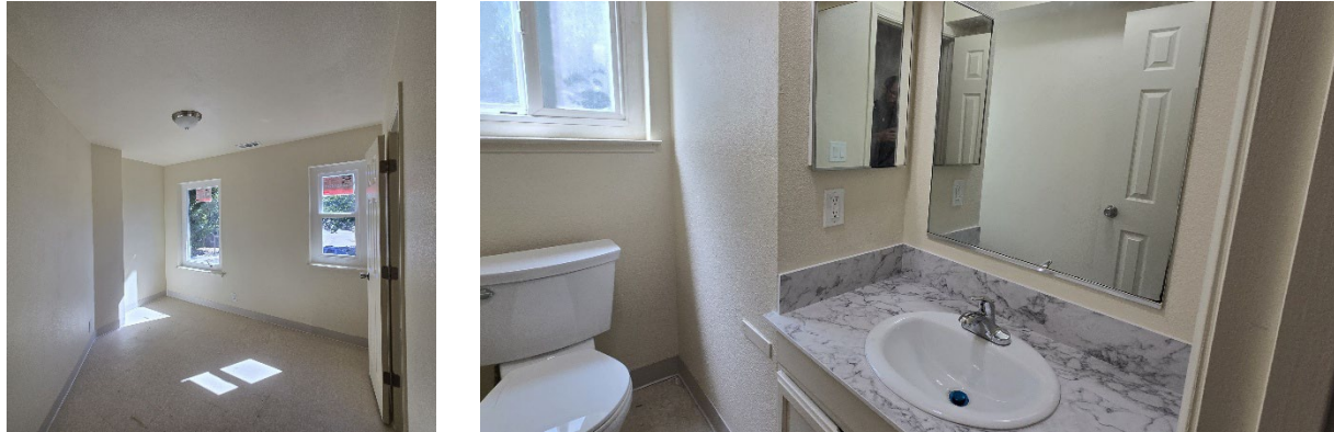
645 Gardella Avenue, Oroville – Fire restoration (Project Complete)
