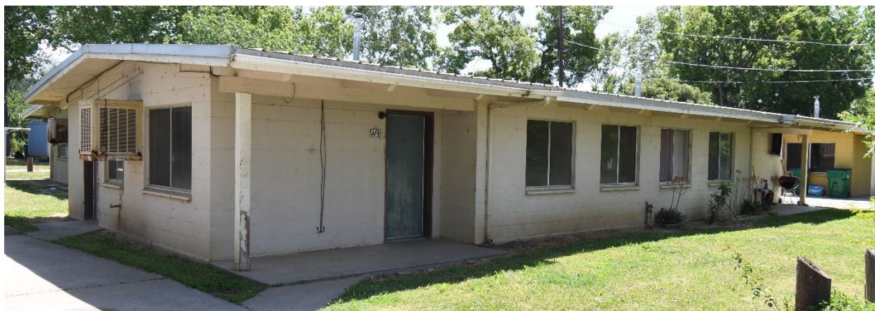
Unrenovated 1980's era Concrete-block Unit
