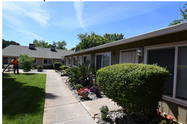
Park Place Apartments, 2105 Park Avenue, Oroville
