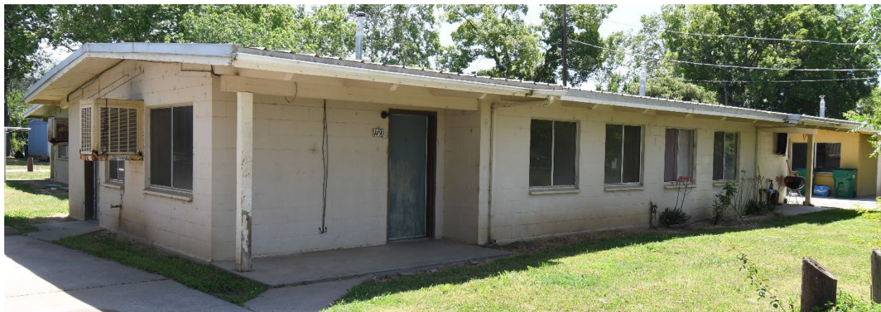
Unrenovated 1980's era Concrete-block Unit
