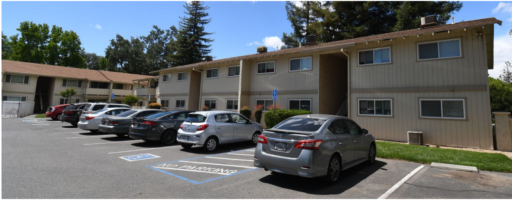
Alamont Apartments, 811 West East Avenue, Chico
