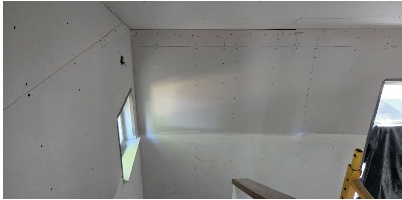
645 Gardella Avenue, Oroville (rehabilitation in process)
