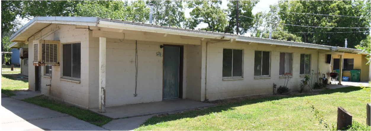
Unrenovated 1980's era Concrete-block Unit
