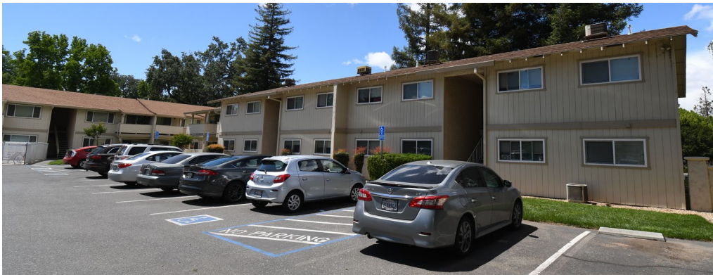
Alamont Apartments, 811 West East Avenue, Chico
