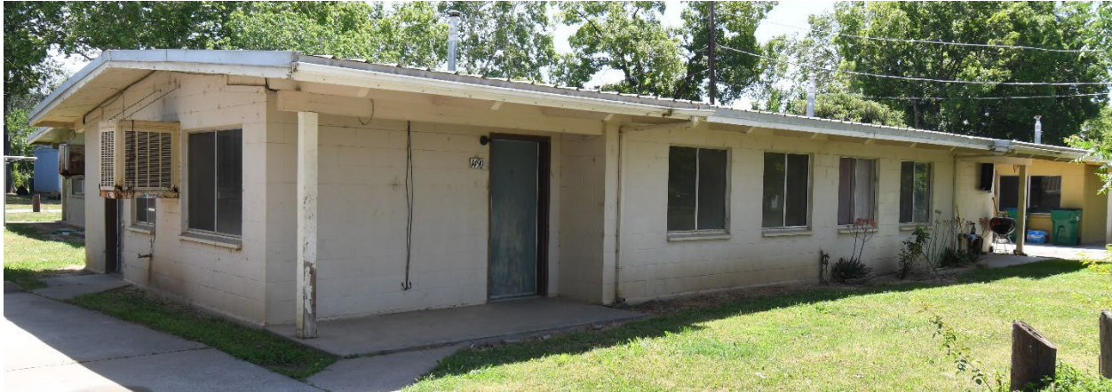
Unrenovated 1980's era Concrete-block Unit
