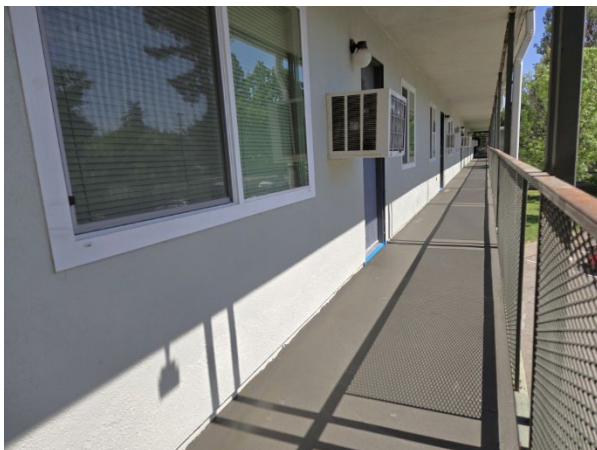
First coat of deck coating system installed
