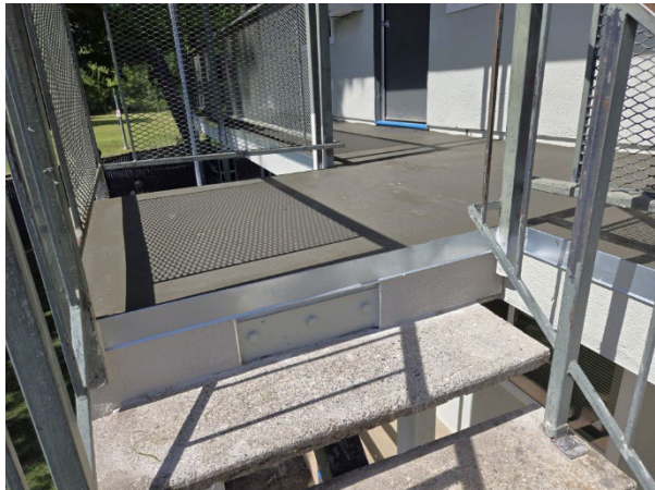
First coat of deck coating system installed at landing
