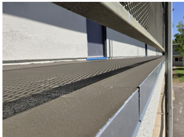
Edge flashing and first coat of deck coating system
