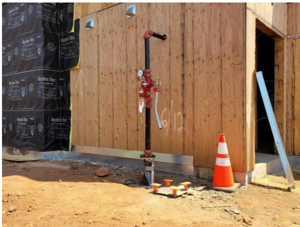
Fire sprinkler riser in place
