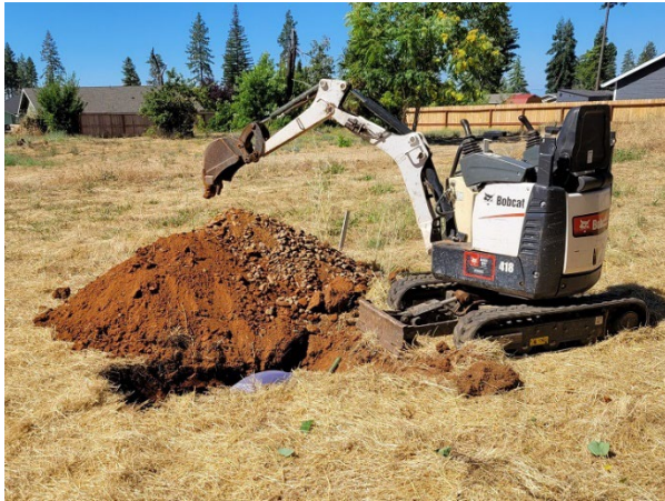
Repair to leach line in progress
