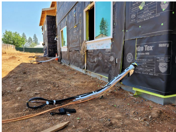
HVAC line set in place
