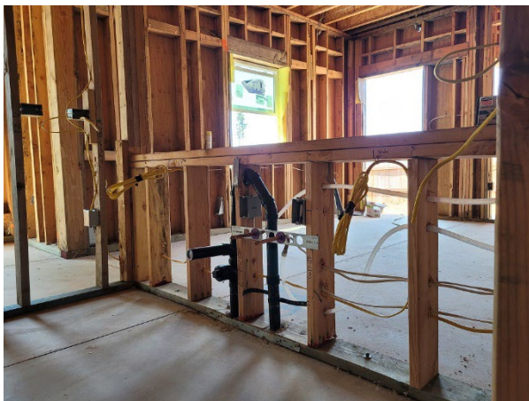
Plumbing and electrical rough-in complete
