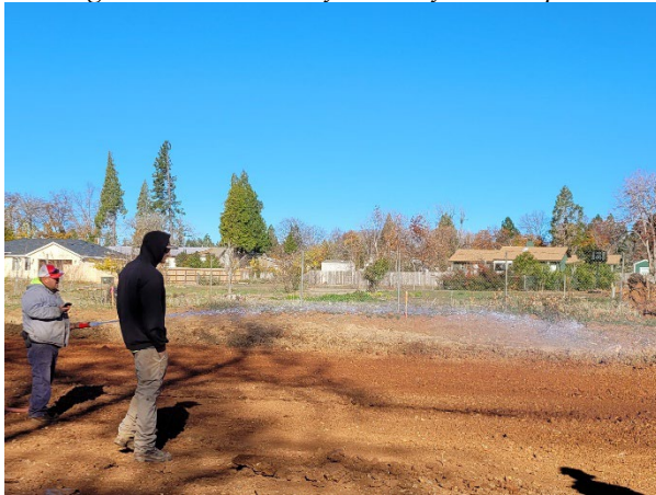
Grading activities underway at Kathy Court Apartments
