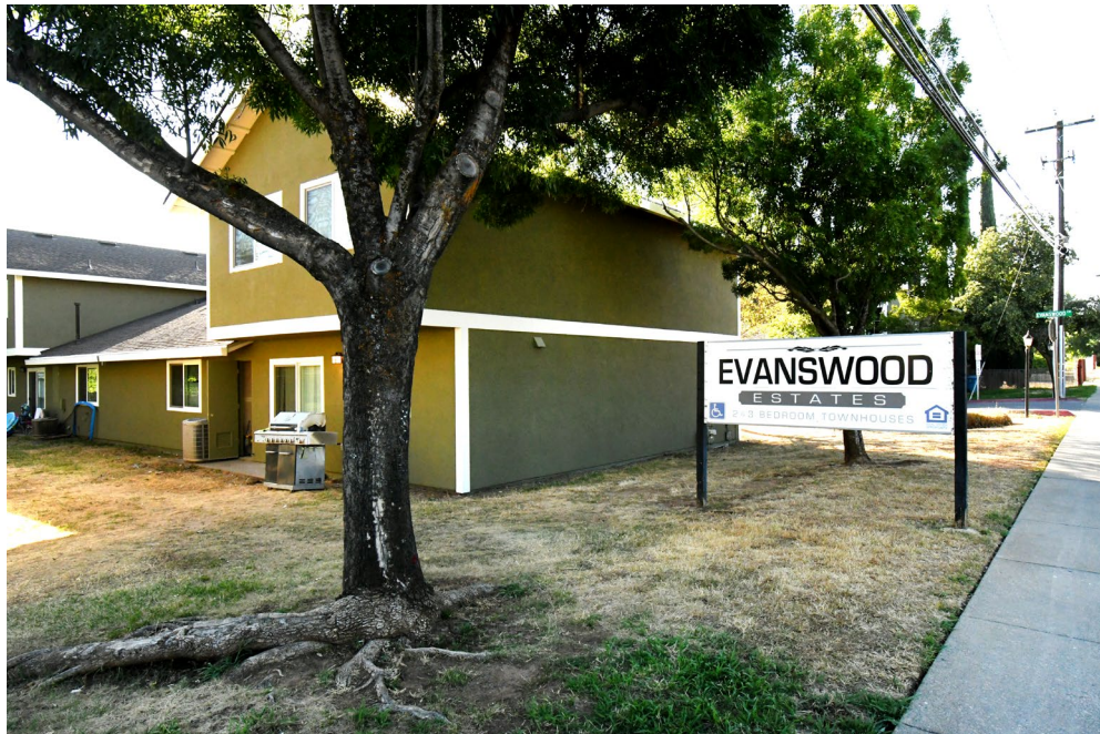
Evanswood Estates, Table Mountain Boulevard, Oroville - new façades.
