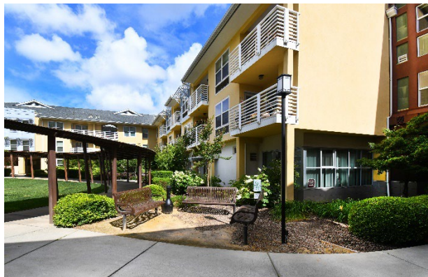
1200 Park Avenue Apartments, Chico
