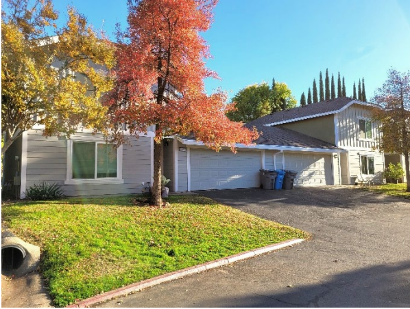
Completed exterior improvements at Evanswood Estates
