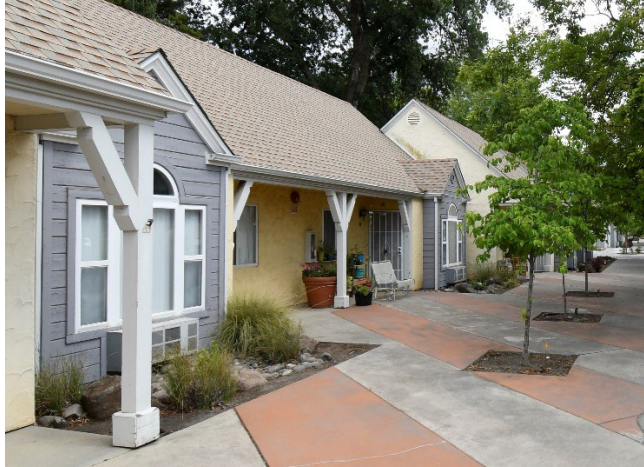
Walker Commons Apartments, 678 Buttonwillow Lane, Chico
