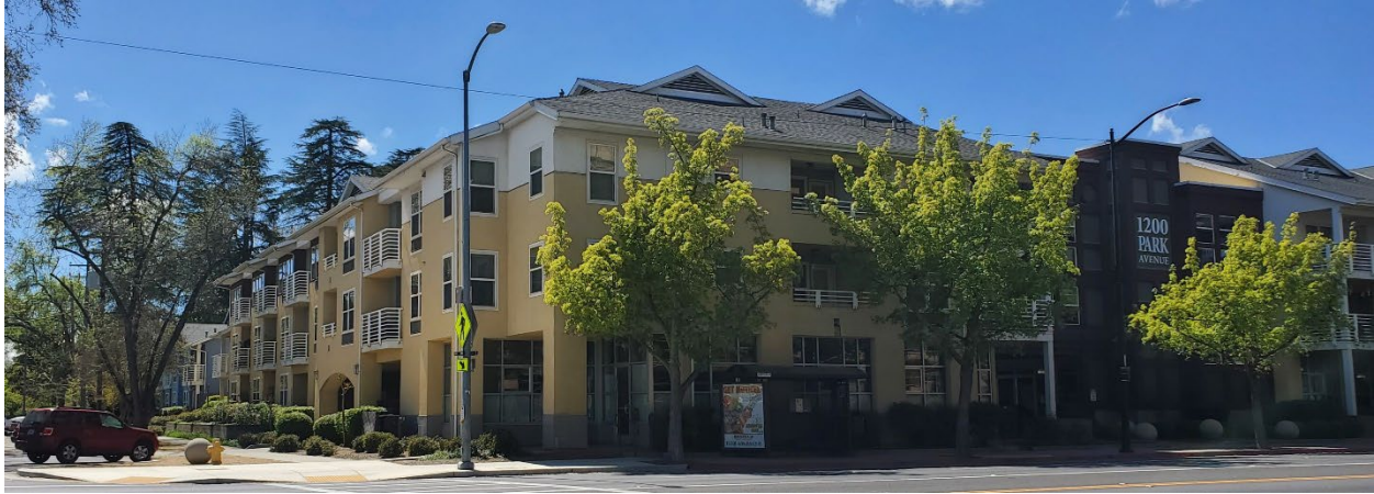
1200 Park Avenue Apartments, Chico
