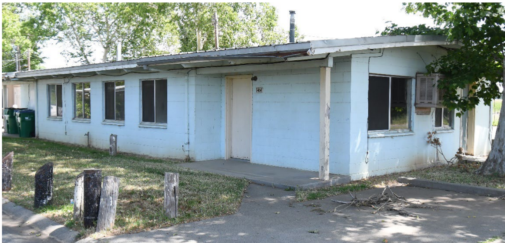
Unrenovated 1980’s era Concrete Block Unit
