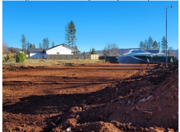
Grading activities underway at Kathy Court Apartments
