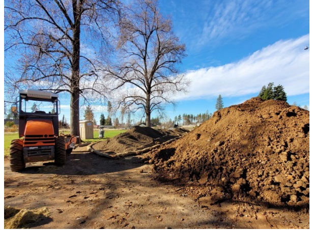
Grading activities underway at Kathy Court Apartments
