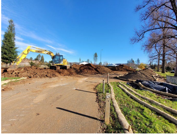
Grading activities underway at Kathy Court Apartments
