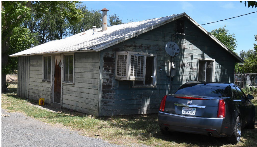
1930’s era Wood Frame Unit
