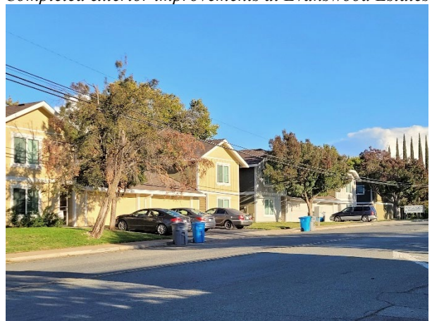
Completed exterior improvements at Evanswood Estates
