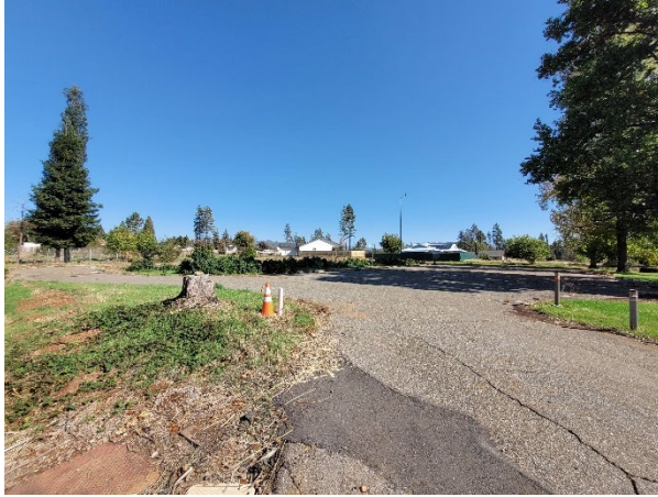
Kathy Court Apartments prior to reconstruction
