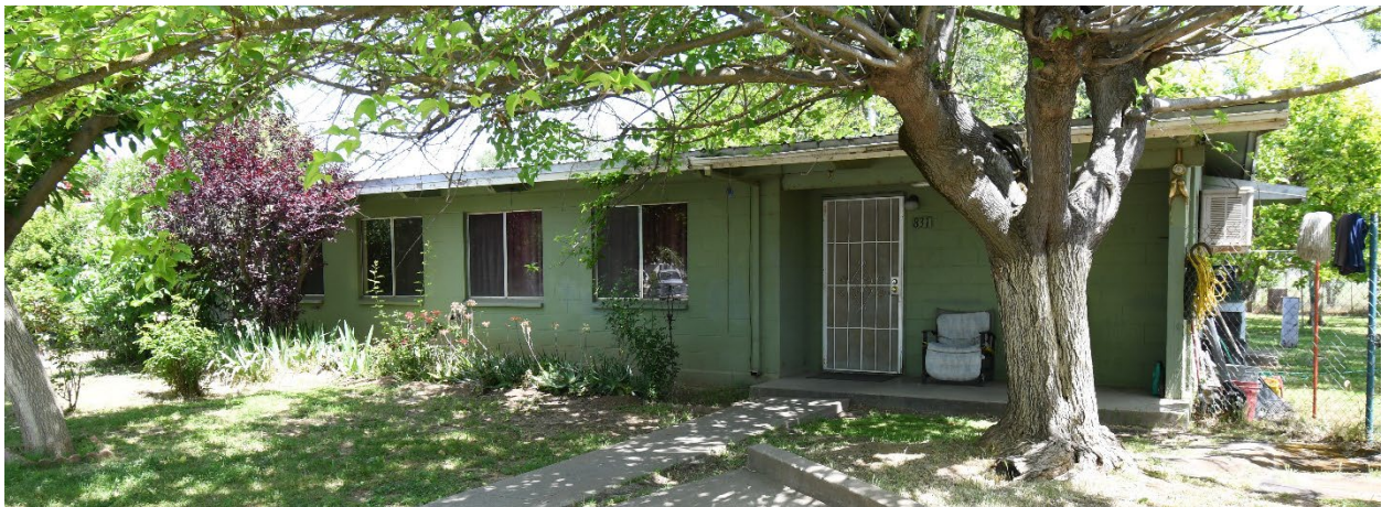
Unrenovated 1980's era Concrete Block Unit
