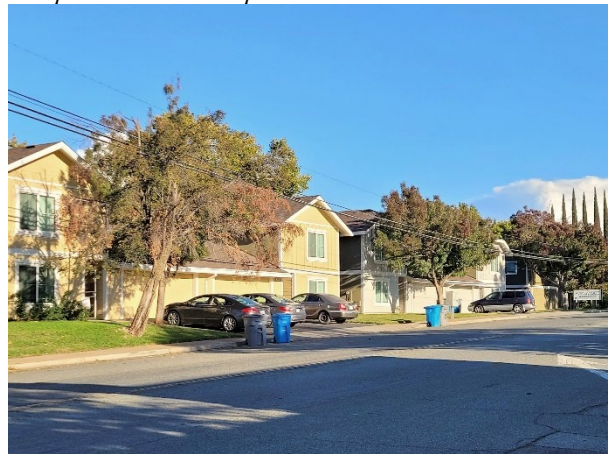
Completed exterior improvements at Evanswood Estates
