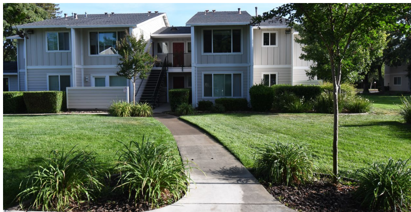
Gridley Springs Apartments II, 210 Ford Avenue, Gridley
