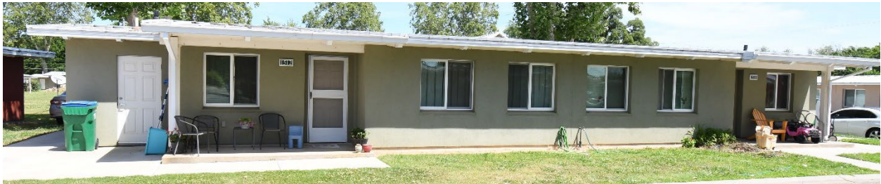
Renovated 1980's era housing
