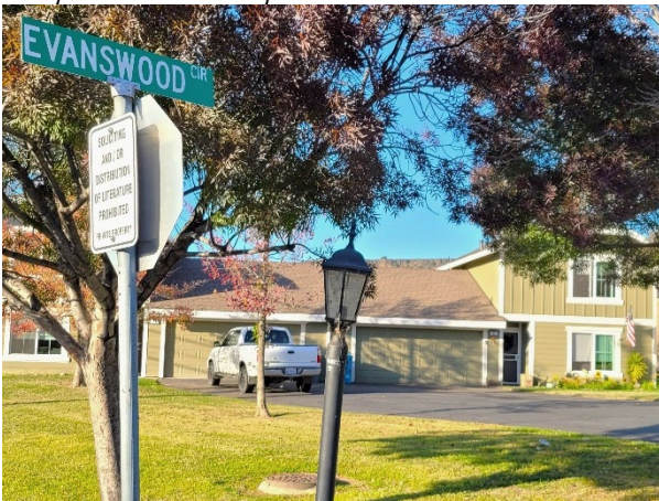
Completed exterior improvements at Evanswood Estates
