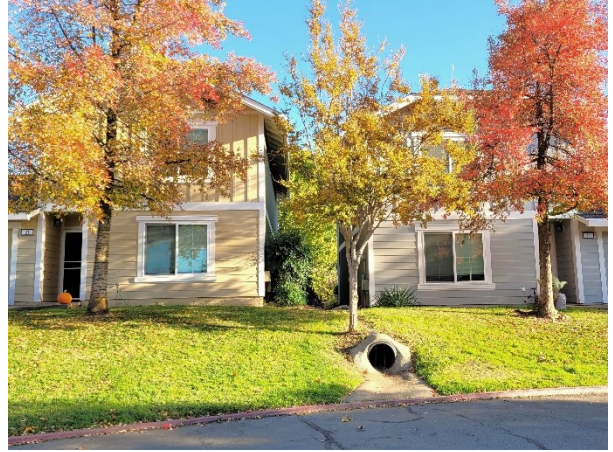
Completed exterior improvements at Evanswood Estates
