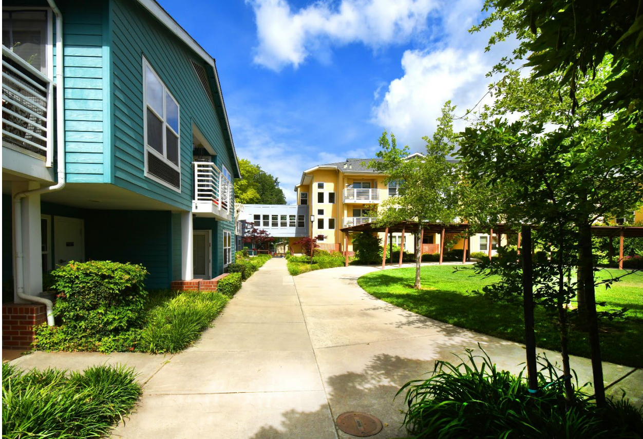
1200 Park Avenue Apartments, Chico
