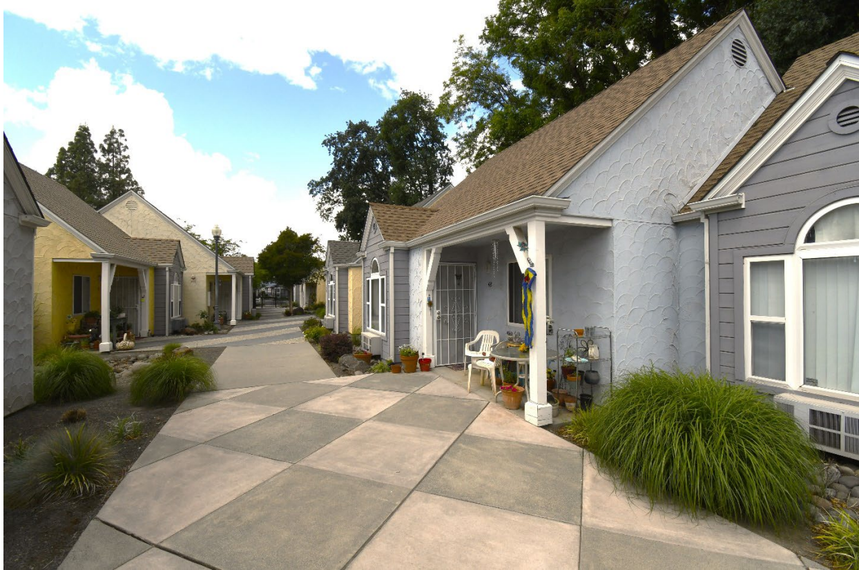
Walker Commons Apartments, 678 Buttonwillow Lane, Chico
