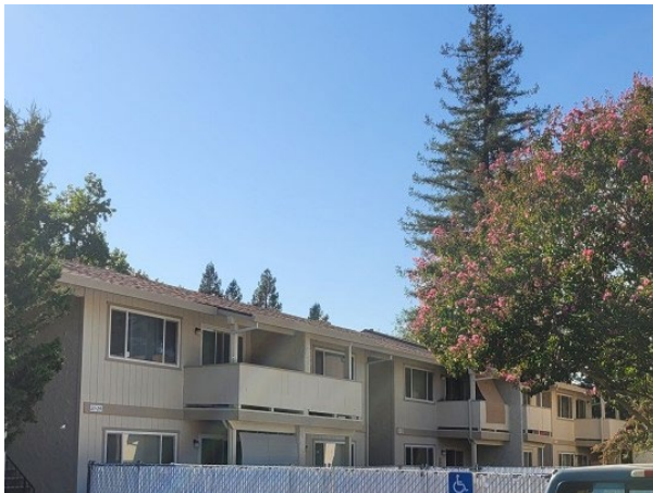
Completed balcony replacement at Alamont Apartments
