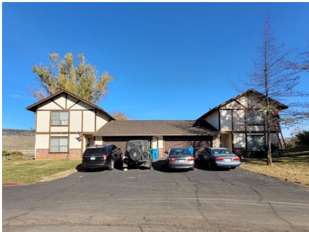
Unit 37 and 41 before improvements
