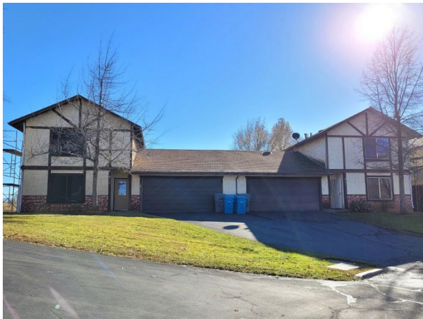
Unit 21 and 25 before improvements
