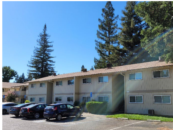
Completed roof replacement at Alamont Apartments
