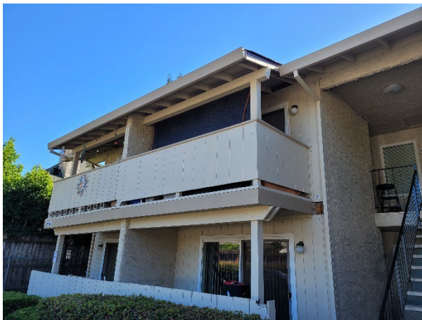
Completed balcony replacement at Alamont Apartments
