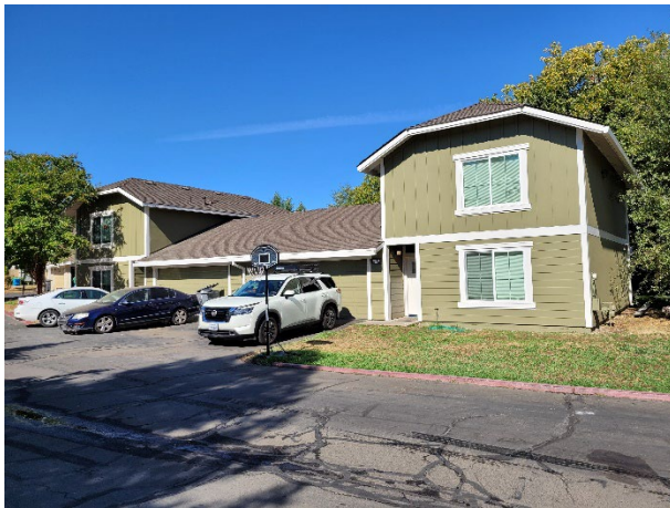
Completed exteriors: Units 12/16, Evanswood Circle
