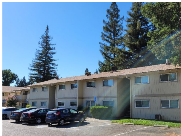
Completed roof replacement at Alamont Apartments
