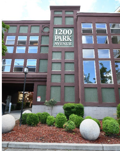
1200 Park Avenue Apartments, Chico
