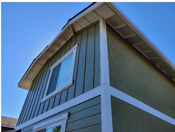
Completed exterior: Unit 36, Evanswood Circle
