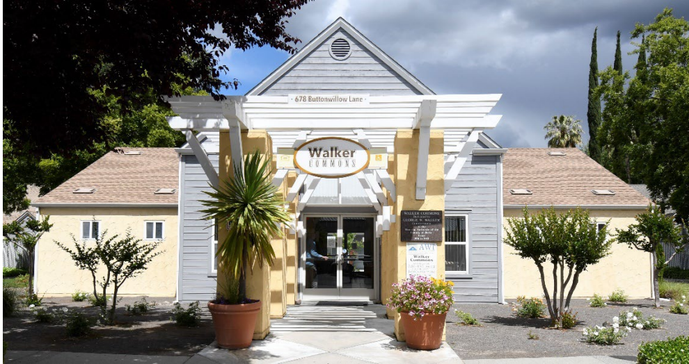
Walker Commons Apartments, 678 Buttonwillow Lane, Chico
