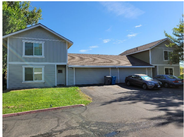
Completed exteriors: Units 41/45, Evanswood Circle
