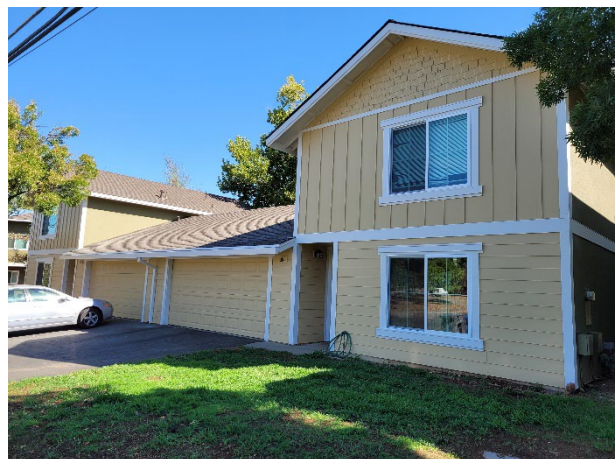
Completed exterior: Unit 364 Table Mtn. Blvd.
