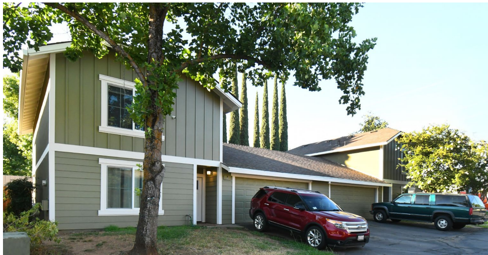
Evanswood Estates, Table Mountain Boulevard, Oroville - new façades
