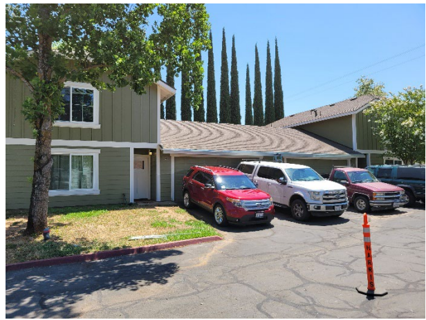
Completed exterior improvements at unit 5 and 9
