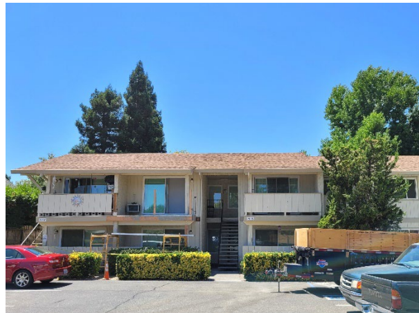
Completed balcony replacement at Alamont Apartments
