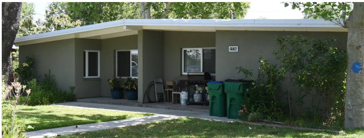
Renovated 1980's era housing
