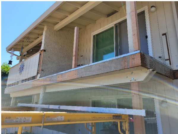
Completed balcony replacement at Alamont Apartments
