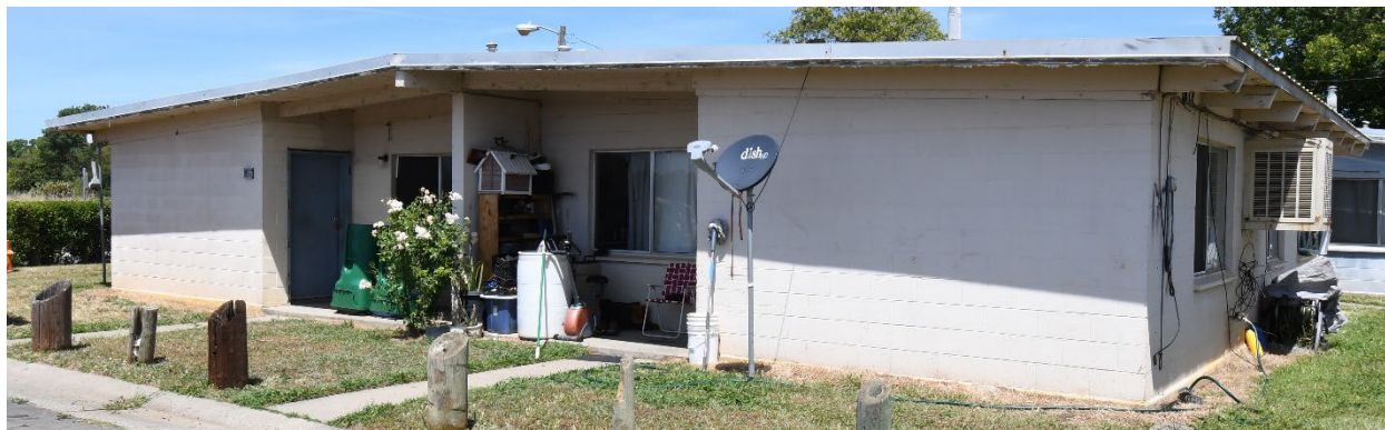
1980's-era Concrete Block duplex unit – unrenovated
