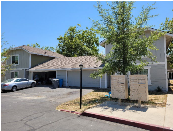
Completed exterior improvements at unit 28 and 32
