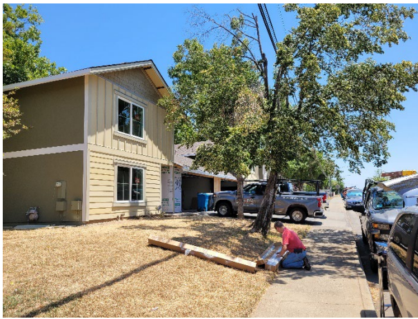
Exterior siding installation nearly complete at Unit 368
