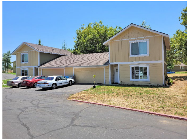
Completed exterior improvements at unit 20 and 24
