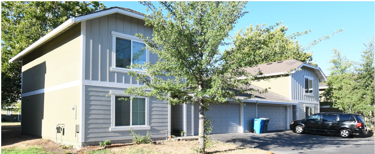
Evanswood Estates, Table Mountain Boulevard, Oroville - new façades
