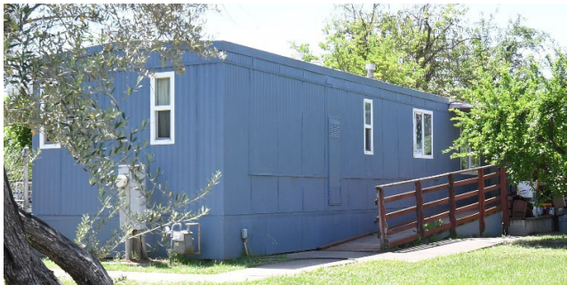
Trailer Unit – East Gridley Road
