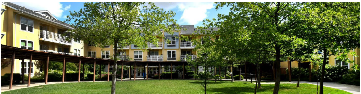
Inner Courtyard, 1200 Park Avenue Apartments, Chico
