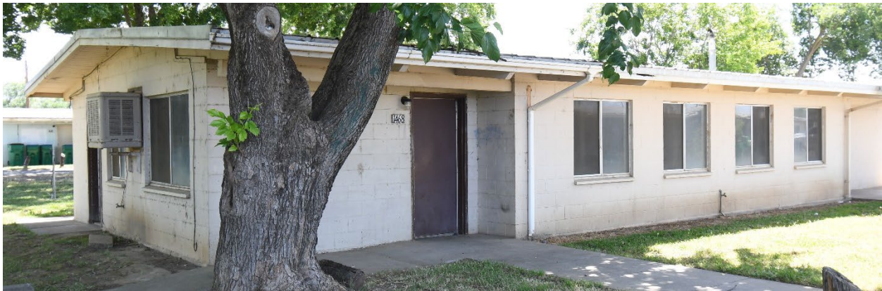
1980's-era Concrete Block duplex unit – unrenovated
