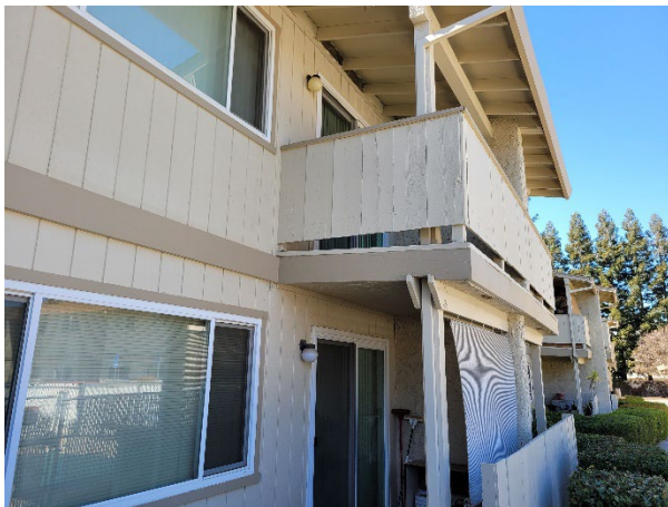
Completed balcony replacement at Alamont Apartments
