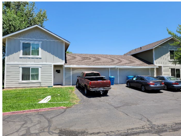
Completed exterior improvements at unit 37 and 41
