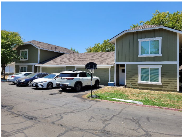
Completed exterior improvements at unit 12 and 16
