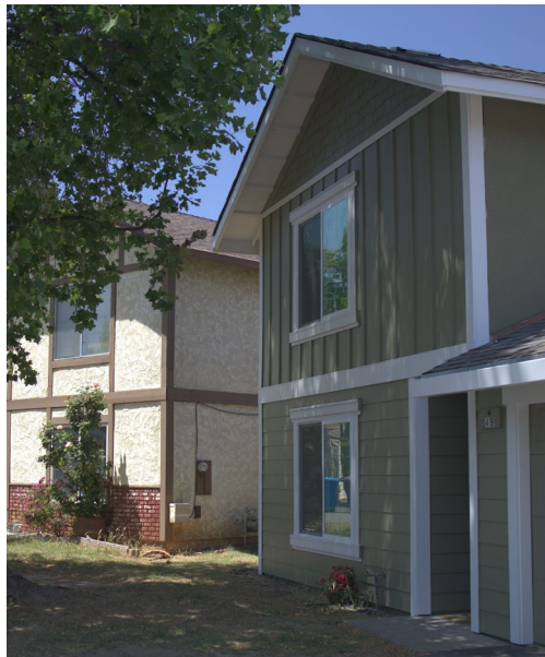
Evanswood Estates – old and new façades
