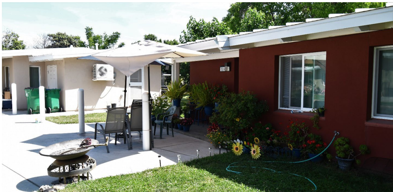
Renovated 1980's era housing
