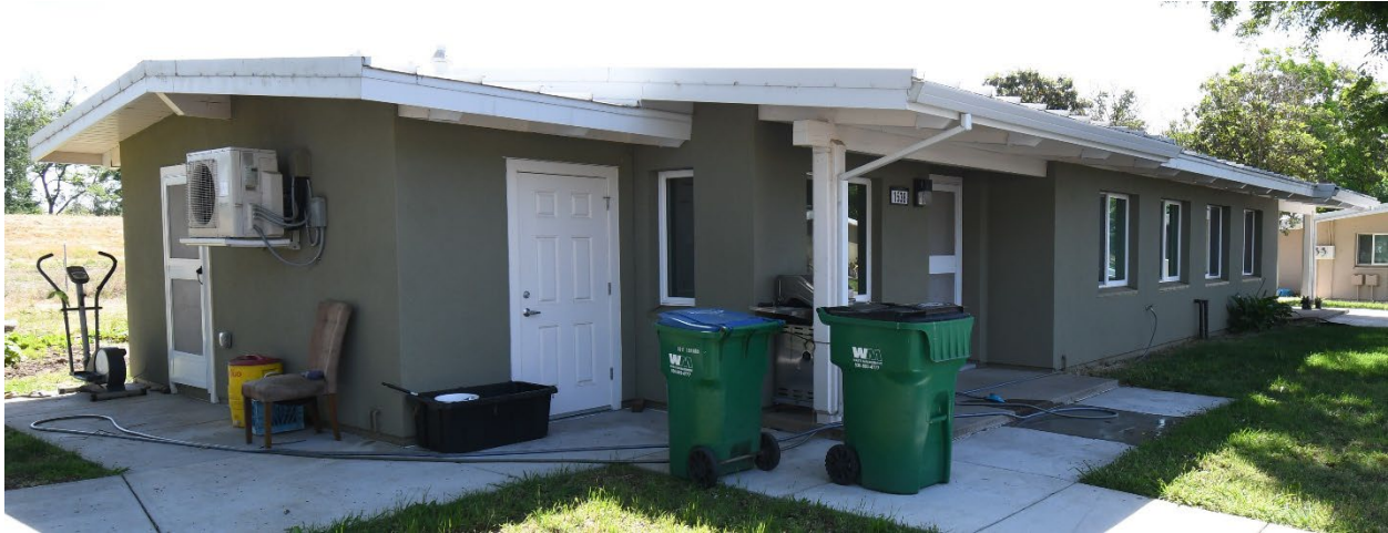
1980's-era Concrete Block unit – renovated
