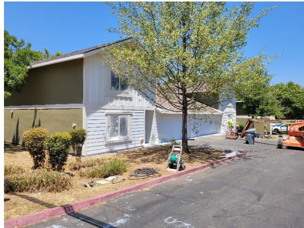
Exterior painting in progress at unit 4
