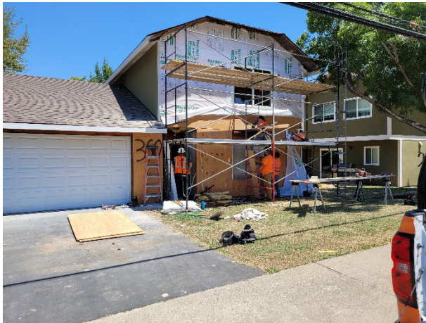
Exterior siding installation in progress at unit 360
