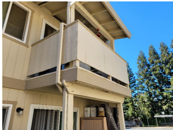
Completed balcony replacement at Alamont Apartments
