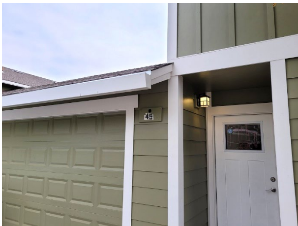
New entry door and exterior lighting installation
