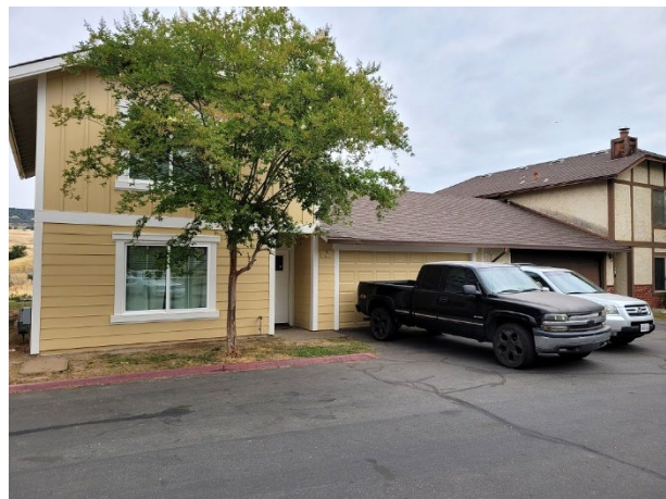
Completed exterior improvements next to unimproved unit
