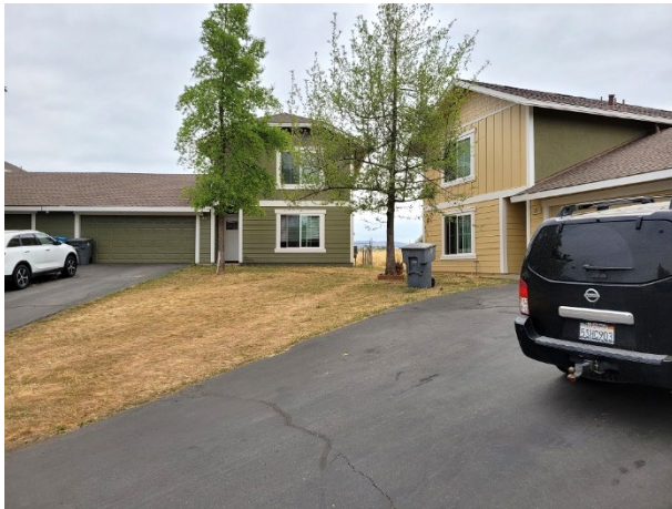
Completed exterior painting at unit 25 & 29
