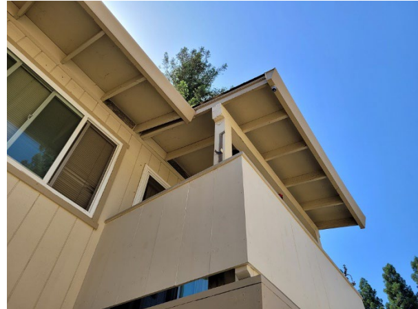
Completed balcony replacement at Alamont Apartments
