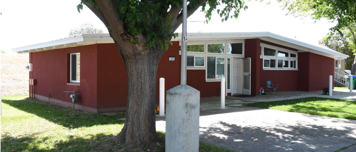
1980's-era Concrete Block duplex unit – renovated
