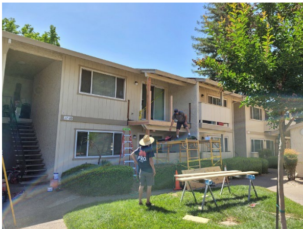
Balcony replacement in process at Alamont Apartments
