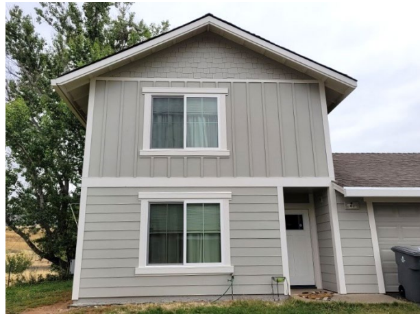
Completed exterior painting at unit 41
