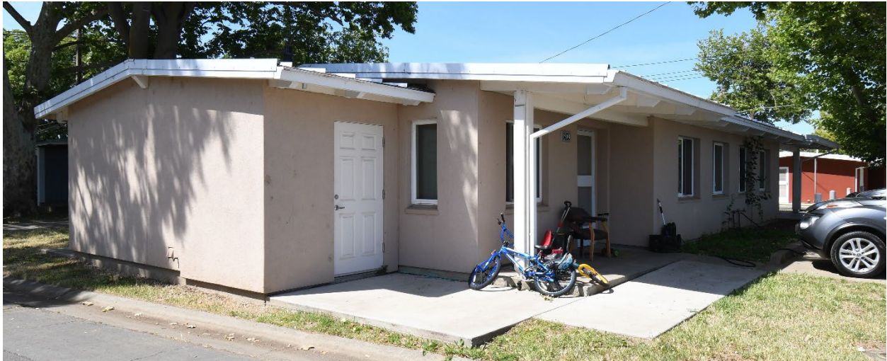
1980's-era Concrete Block unit – renovated
