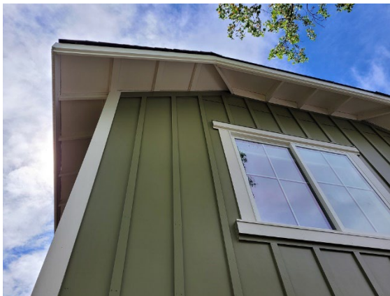
Exterior Painting Detail at Unit 9
