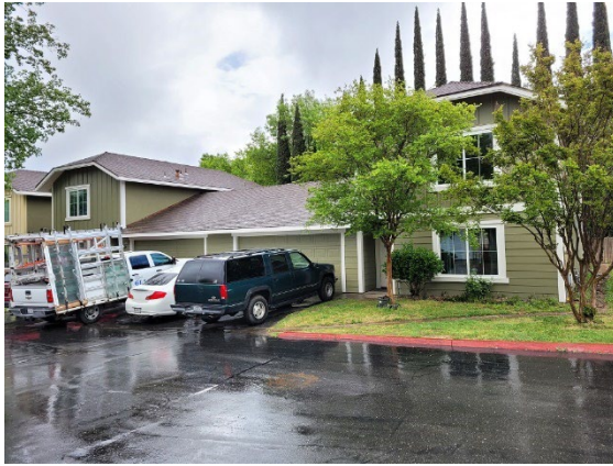
Exterior Painting Complete at Unit 5 & 9
