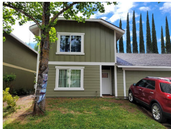
Exterior Painting Complete at Unit 9
