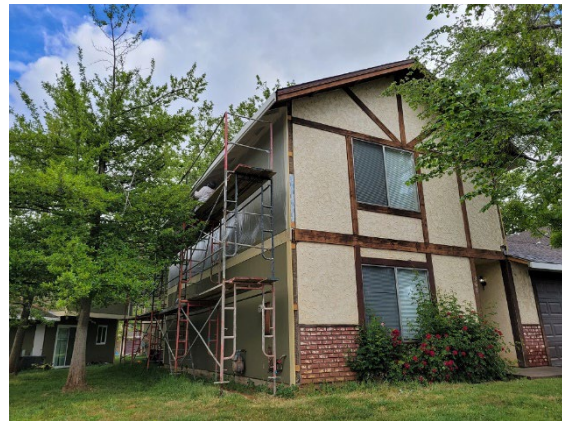
New Trim Installation at Unit 368
