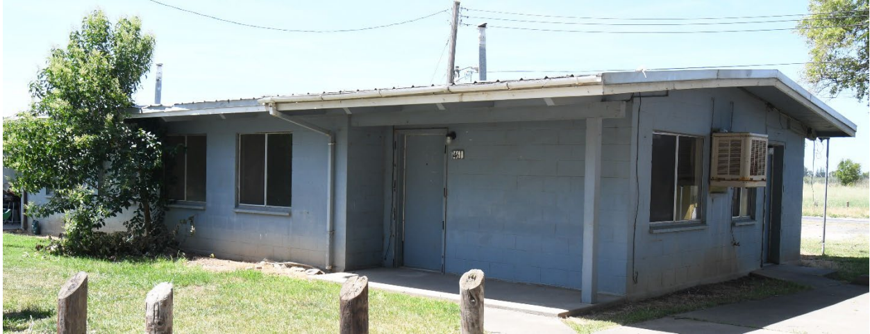
1980's-era Concrete Block unit – unrenovated, unoccupied
