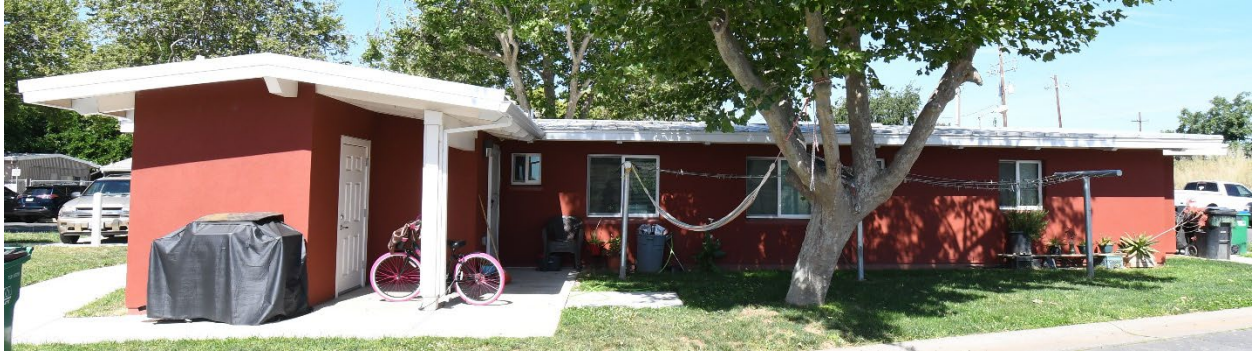
1980's-era Concrete Block duplex unit – renovated
