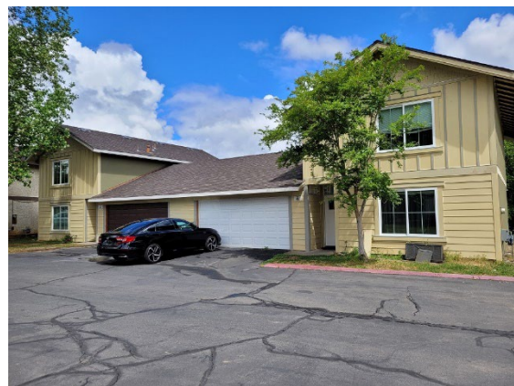
New Siding and Trim Installation at Unit 45 & 49
