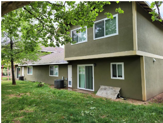
New Window installation at Unit 36
