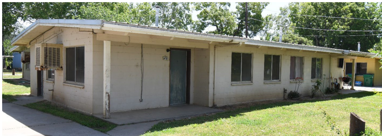
1980's-era Concrete Block unit – unrenovated, unoccupied
