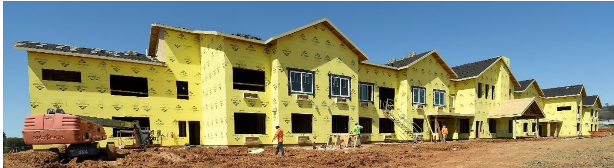
Prospect View Apts, Oroville - framed up, roofing and windows being installed
