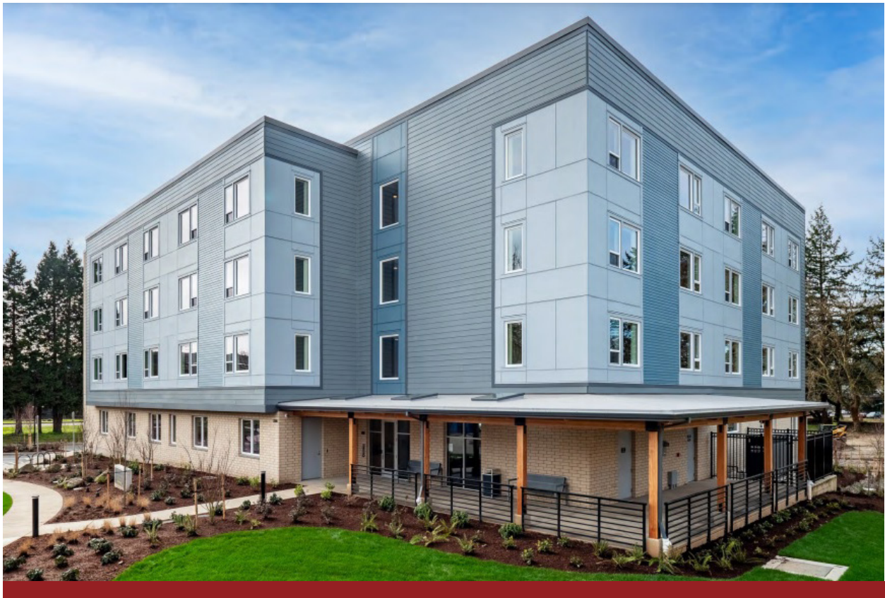
Homes for Good's The Commons on MLK (Ore.).
