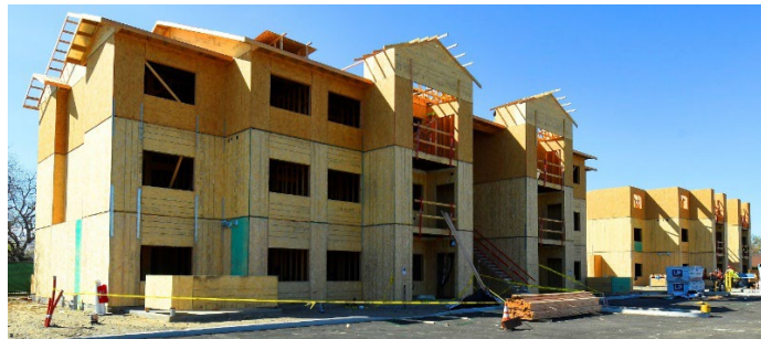
Woodward Apts, Orland – framing well underway.
