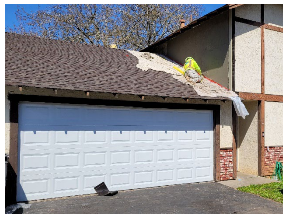
New Garage Door and Stucco Installation at Unit 16
