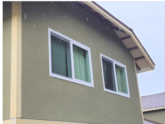
New Rear Window Installation at Unit 5
