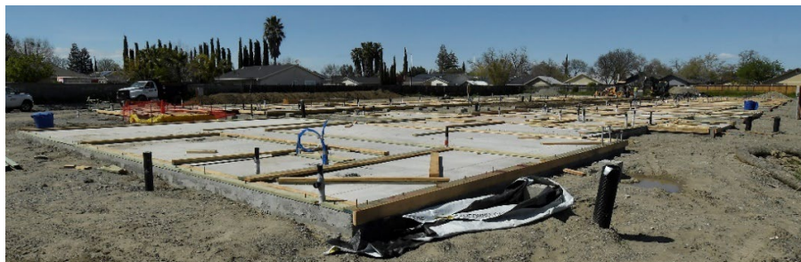
Liberty Bell Apts, Orland – foundations and underground complete, framing has begun.
