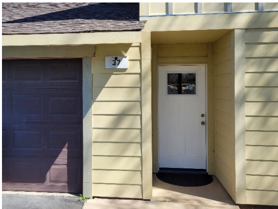
New Entry Door Installation at Unit 37
