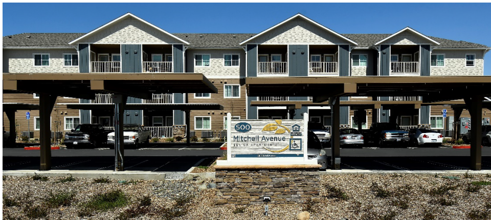
Mitchell Ave Apts I, Oroville – complete and fully occupied
