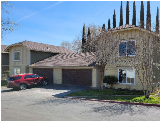
New Siding and Trim Installation at Unit 5
