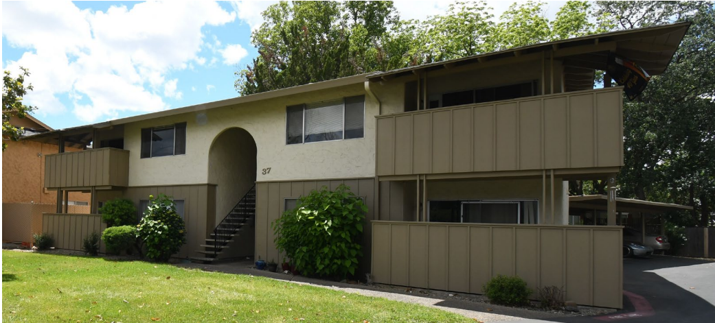
Cordillera Apartments, Cameo Way, Chico
