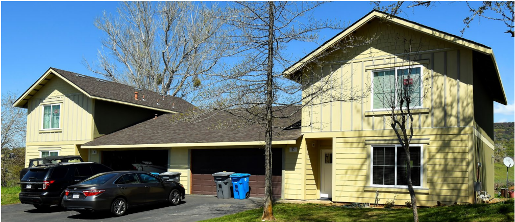
Evanswood Apartments, Table Mountain Boulevard, Oroville – new siding and windows
