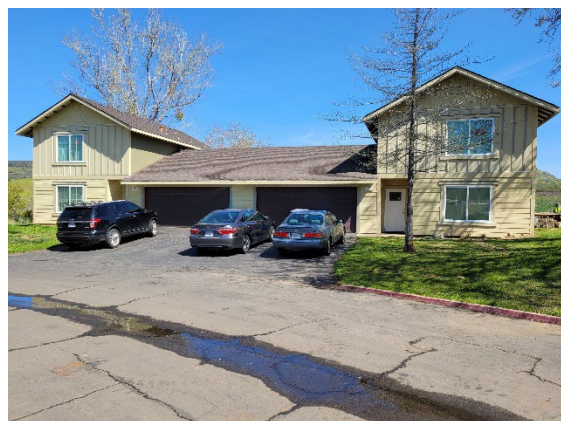
New Siding and Trim Installation at Unit 37 & 41
