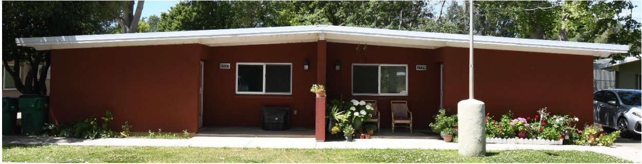
1980's-era Concrete Block duplex unit – renovated
