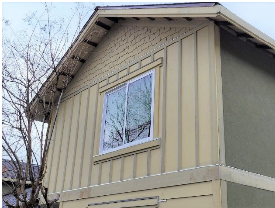
New Siding and Trim Installation at Unit 45
