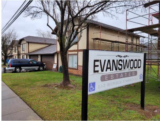
Scaffolding in place near Unit 360
