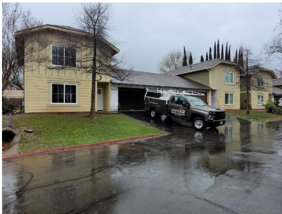
New Siding and Trim Installation at Unit 17
