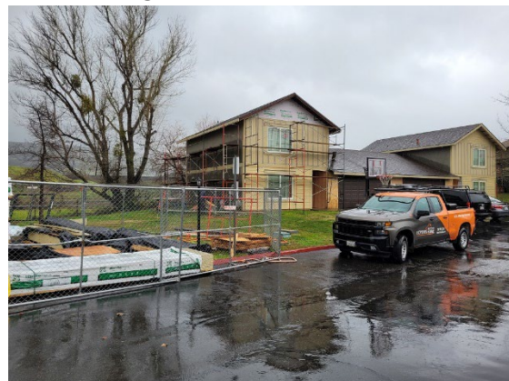
New Siding and Trim Installation at Unit 41
