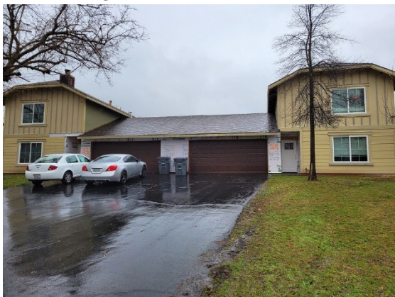
New Siding and Trim Installation at Unit 33
