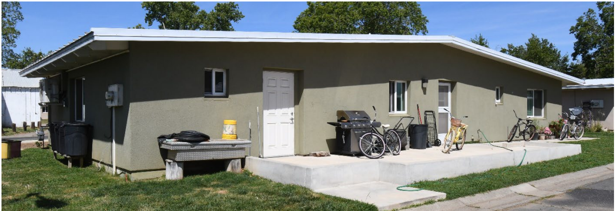
1980's-era Concrete Block unit – renovated
