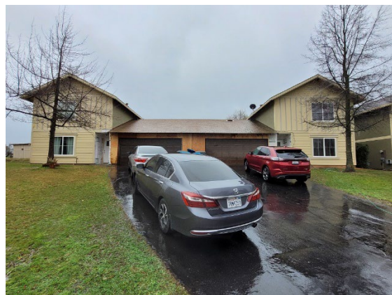
New Siding and Trim Installation at Unit 21
