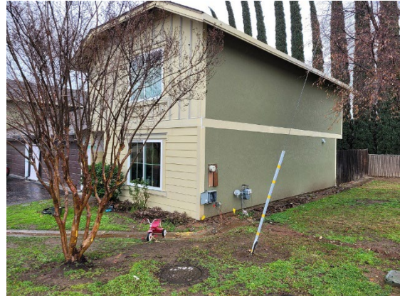
Stucco Color Coat Complete at Unit 5
