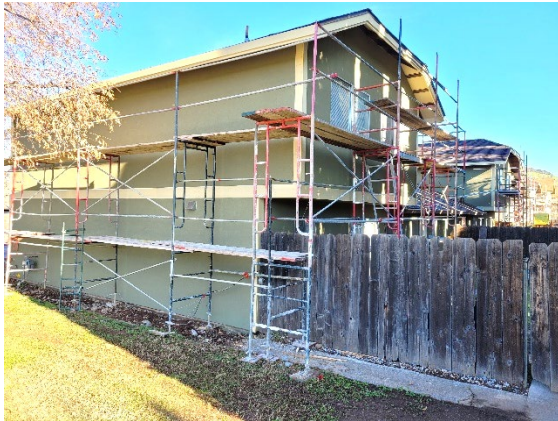
Stucco Color Coat Complete at Unit 5
