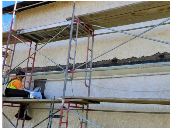
New Trim and Vent Installation at Unit 41
