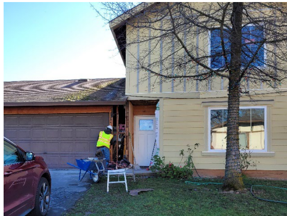
New Siding and Trim Installation at Unit 21
