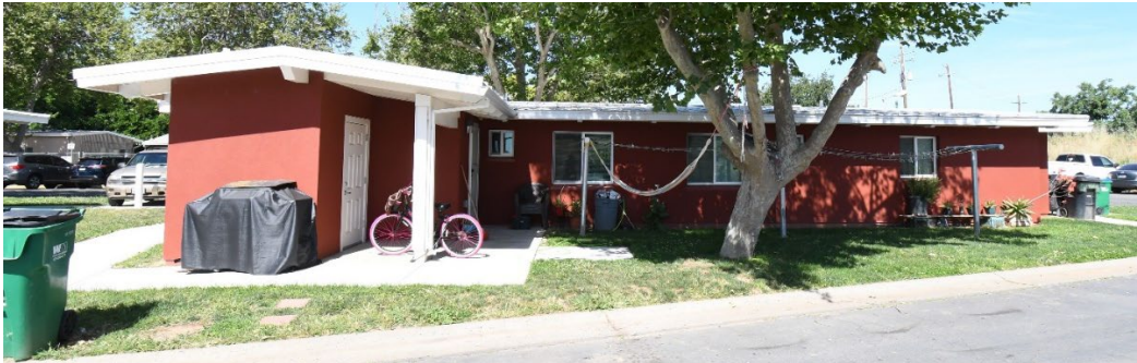
1980's-era Concrete Block unit – renovated
