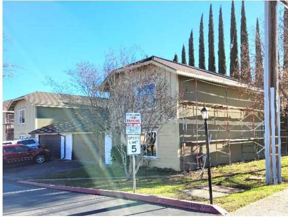
Stucco Color Coat Complete at Unit 5
