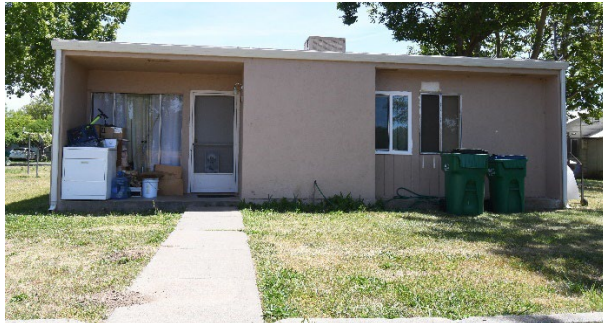
“Demo” unit – State Recycled Materials Demonstration Experiment
