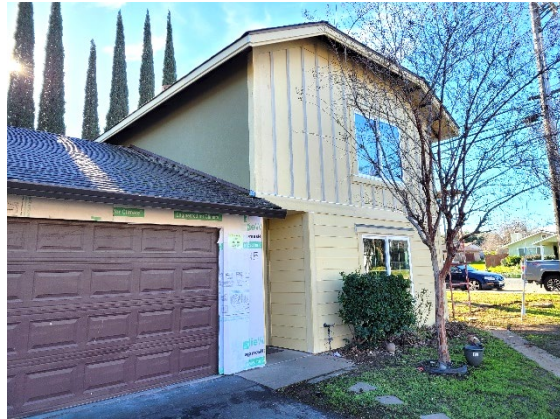
New Siding and Trim Installation at Unit 5
