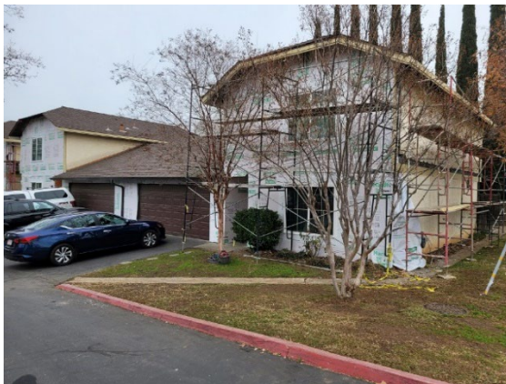
New Siding – scaffolding, siding preparation
